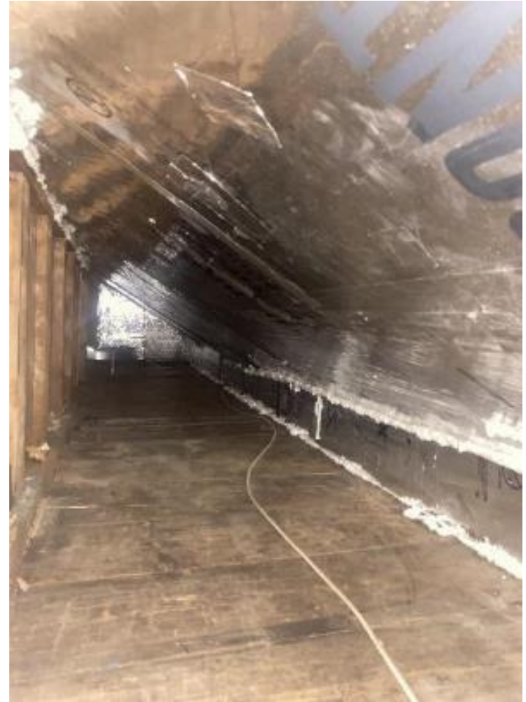
Metal-faced "Thermax" foam board is fire-rated
