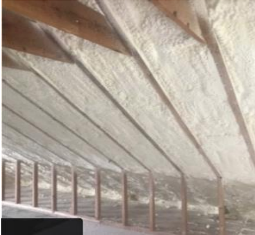
Spray foam prior to drywall fire barrier
