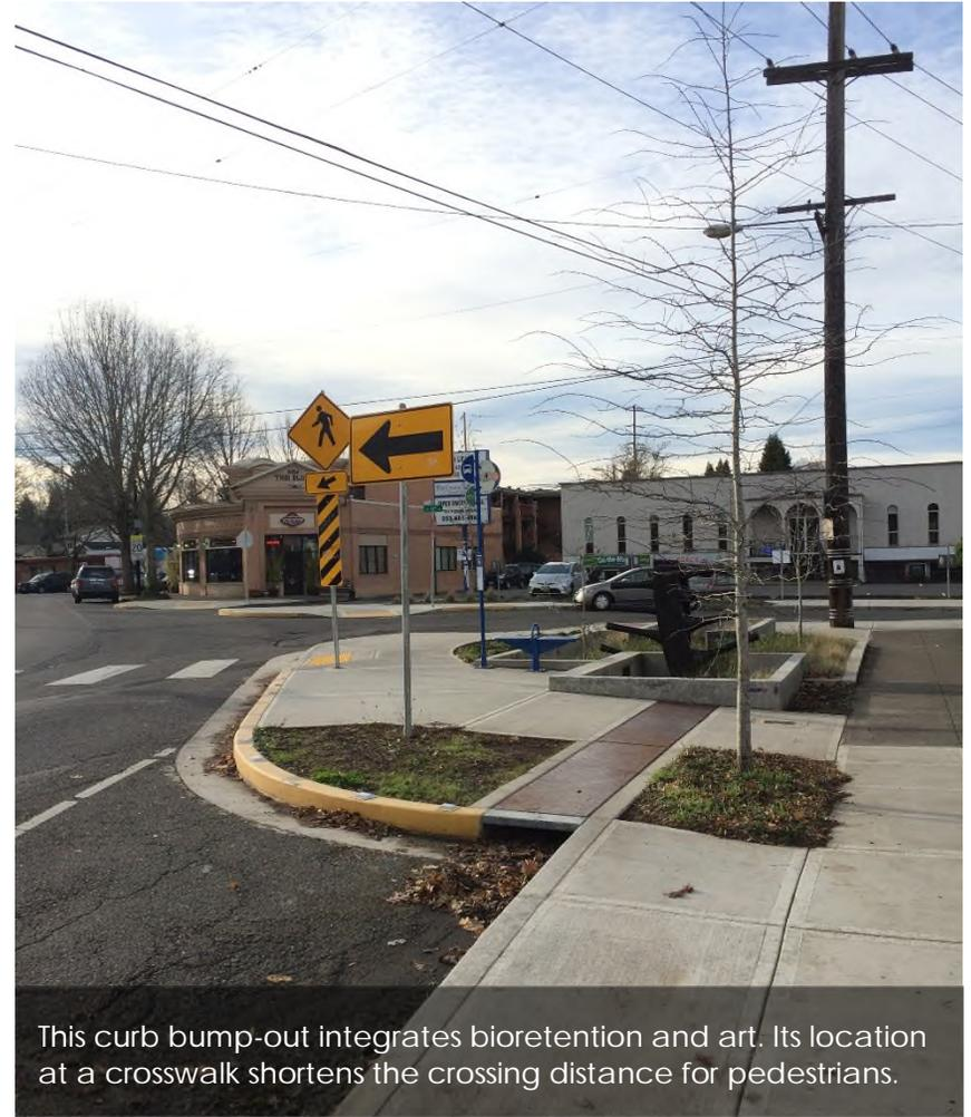
This curb bump-out integrates bioretention and art. Its location at a crosswalk shortens the crossing distance for pedestrians.
