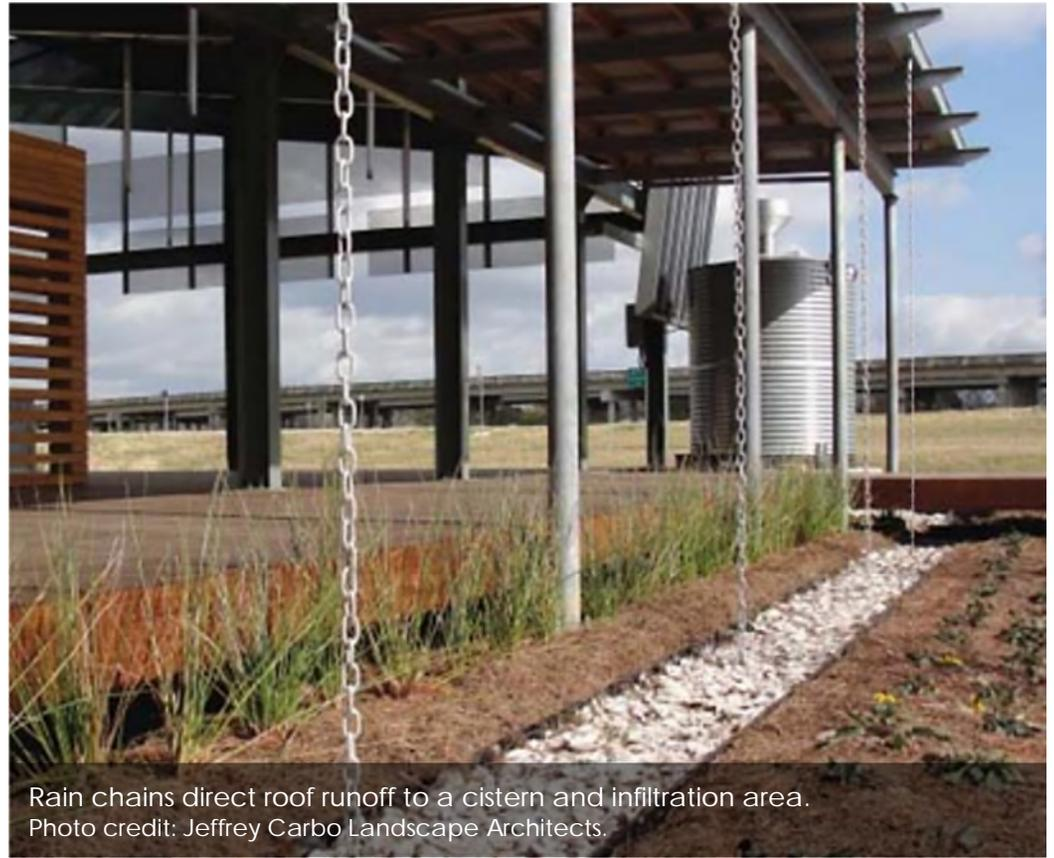
Rain chains direct roof runoff to a cistern and infiltration area.
