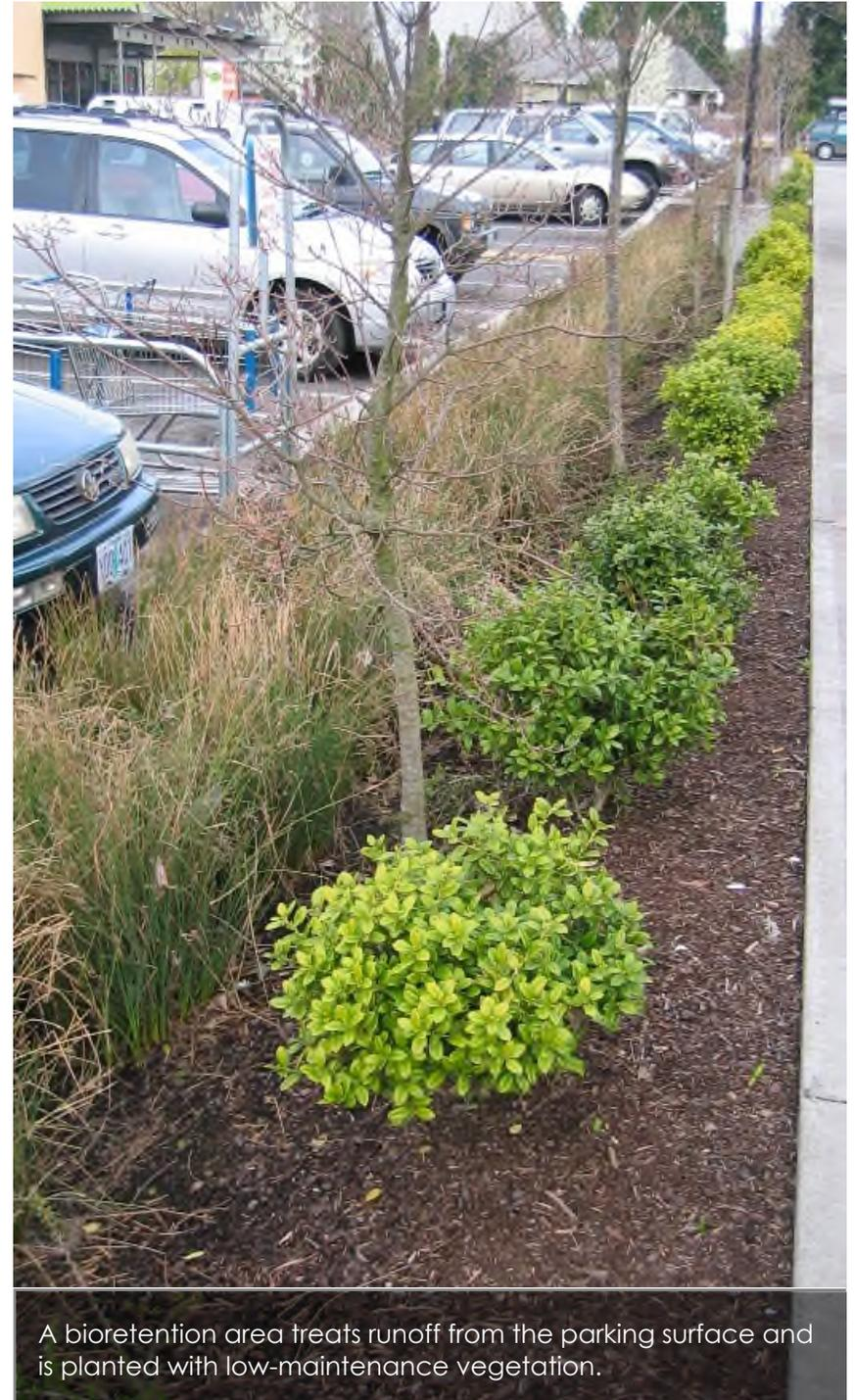
A bioretention area treats runoff from the parking surface and is planted with low-maintenance vegetation.
