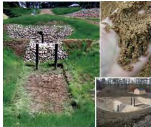
**Figure 5. Sand Filter (Credit: UNHSC)**
