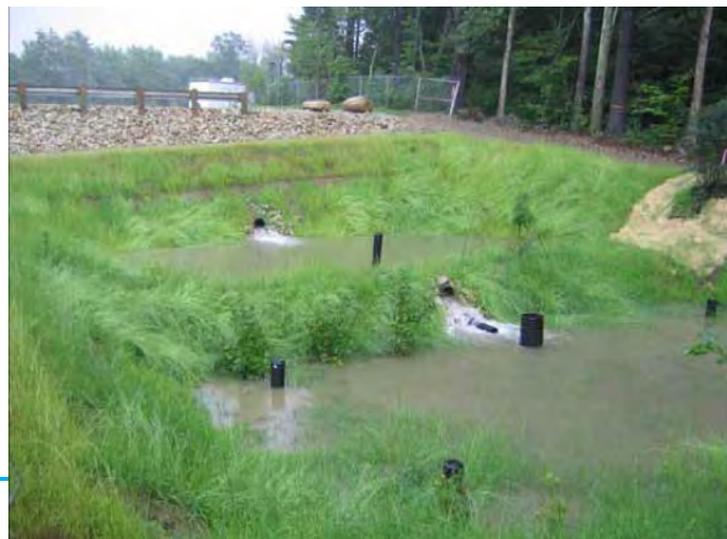
Figure 3. Gravel Wetland (Credit: UNH Stormwater Center)
