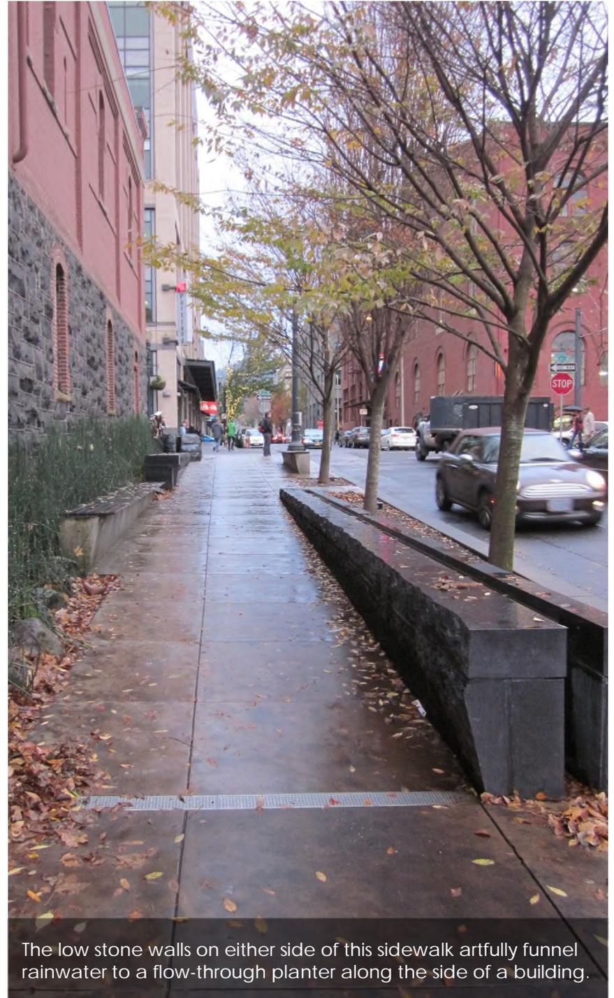
The low stone walls on either side of this sidewalk artfully funnel rainwater to a flow-through planter along the side of a building.
