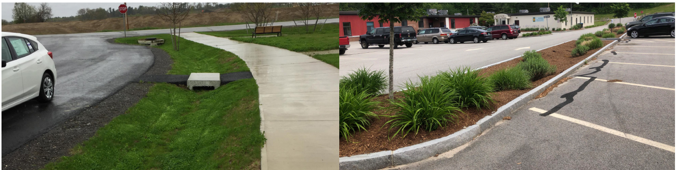
Left: This low impact development bioswale was installed in 2015 as part of the Exeter Subaru expansion that included construction of one part of the small connector roadway between River Road and Market Basket envisioned in the Gateway District. Right: This bioretention system, located at the Stratham Municipal Center, was installed in 2013 as part of a parking lot expansion. This system provides treatment for stormwater runoff carrying pollutants from the parking lots and turf fields and provides clean surface water and groundwater recharge.
