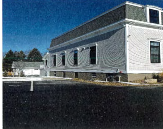
Side (southwest wall)
