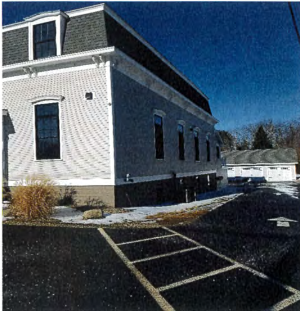
Side (northeast wall)
