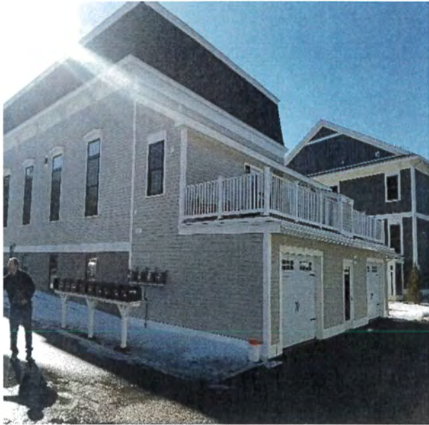
Rear (northwest side)
