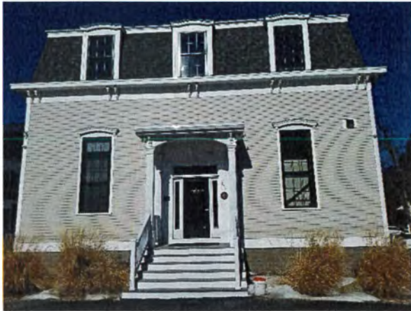
Front (southeast wall)
