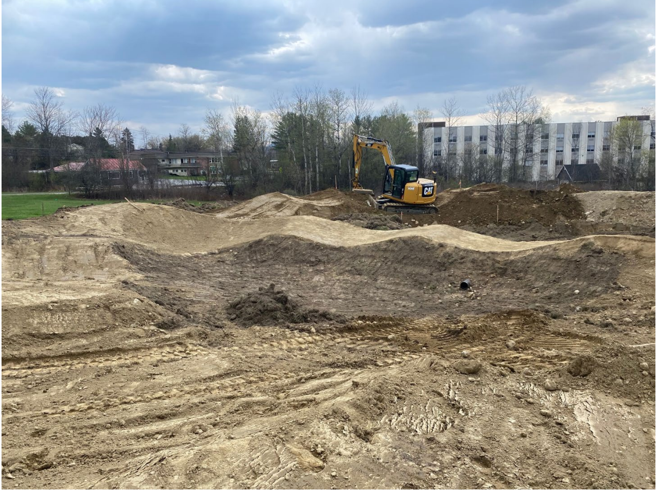
Rutland, VT - under construction.
