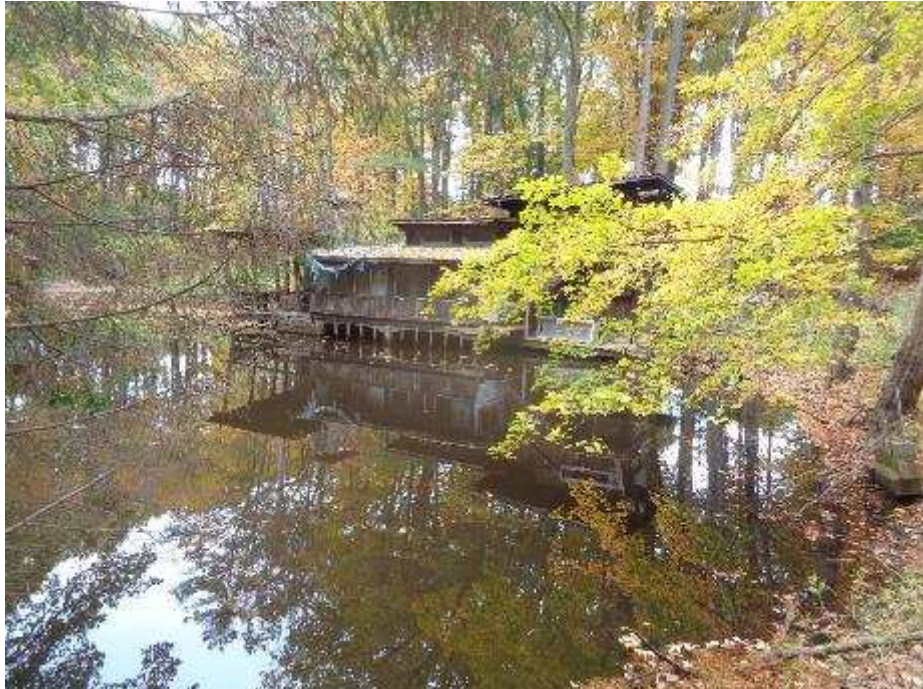
Subject Property – Pond & Camp Building Looking Southeast from Bridge Area - (10/23)
