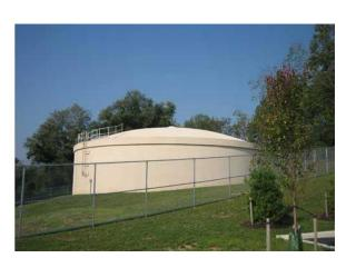
A) Concrete Ground Level Storage Tank
