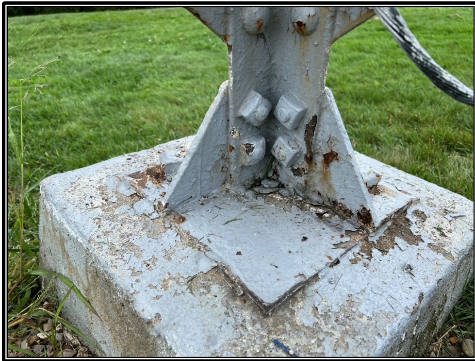
Photo 4: West anchor plate.
