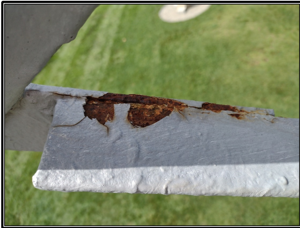
Photo 10: Surface rust at connection.
