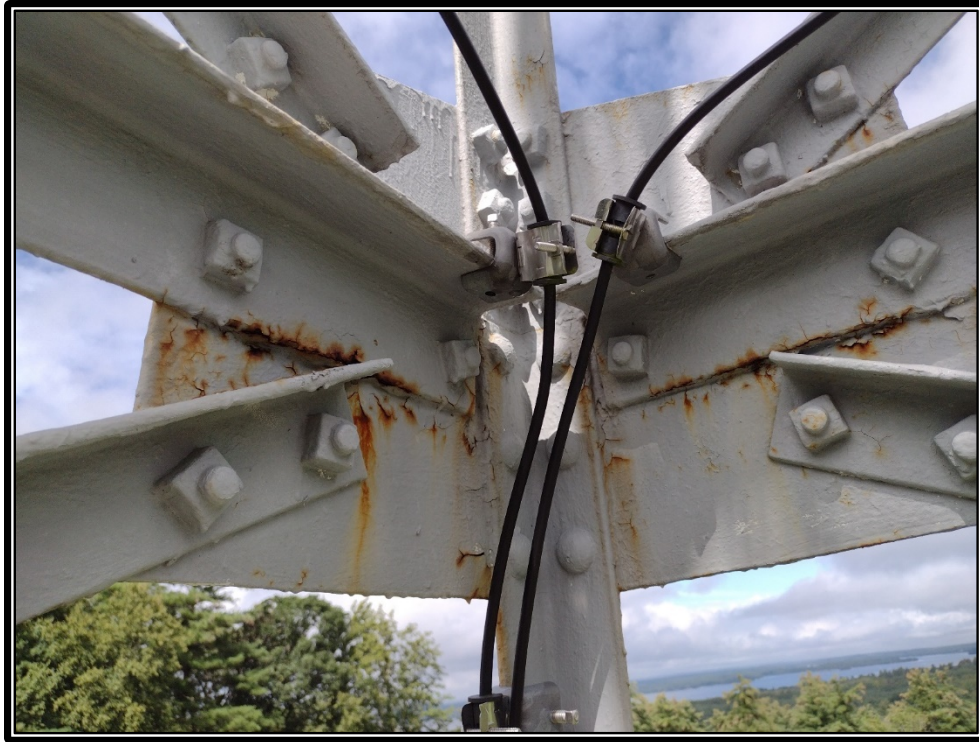
Photo 11: Rust at corner gusset connection.
