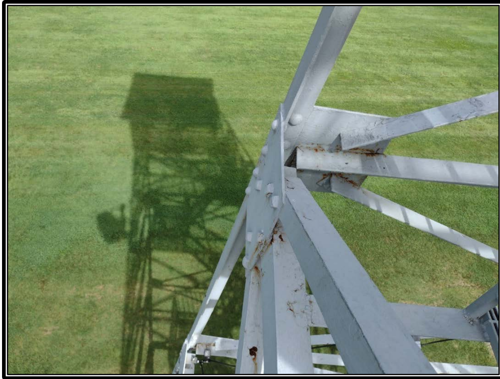
Photo 9: Corner gusset plate connection.
