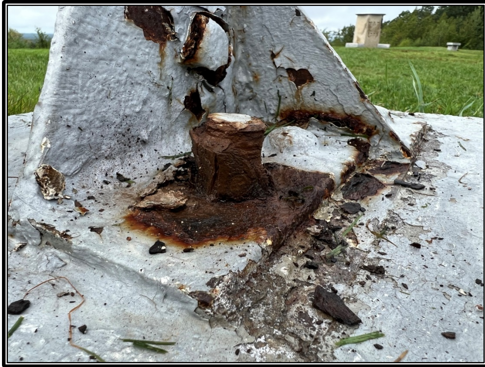
Photo 5: Section loss at north footing anchor rod.
