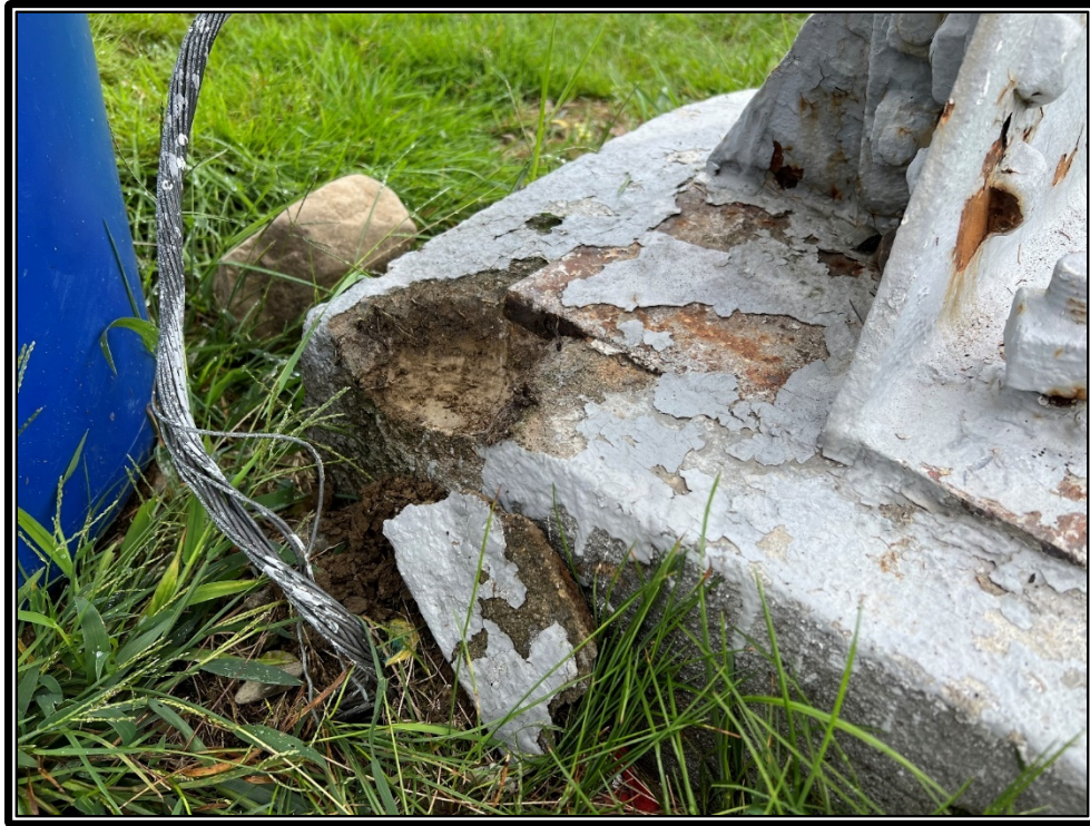
Photo 3: Spall at east footing.
