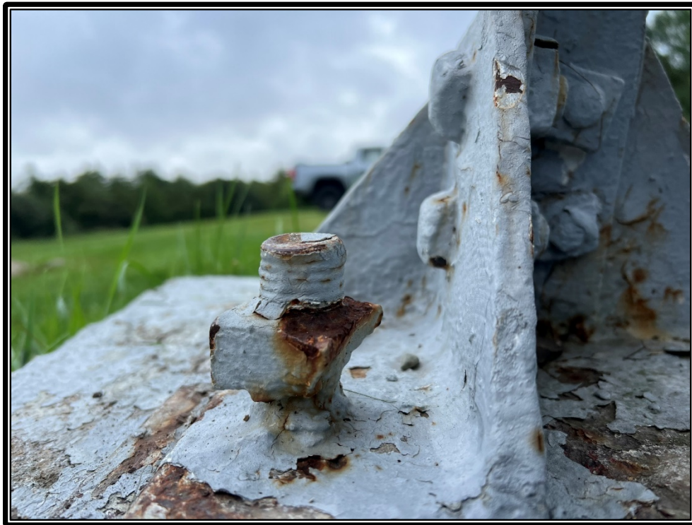
Photo 6: Anchor bolt at east footing.
