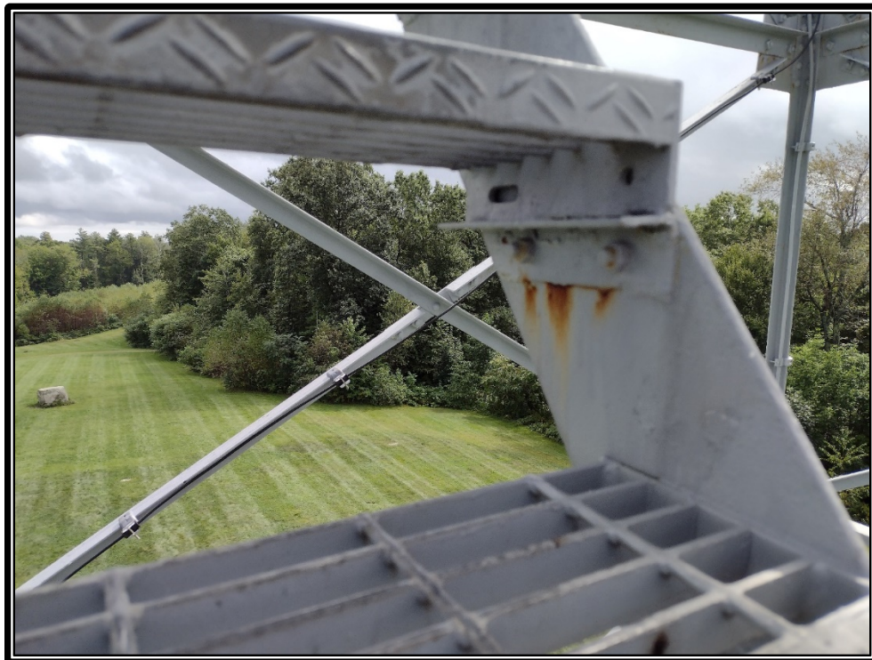
Photo 14: Stair tread connection.
