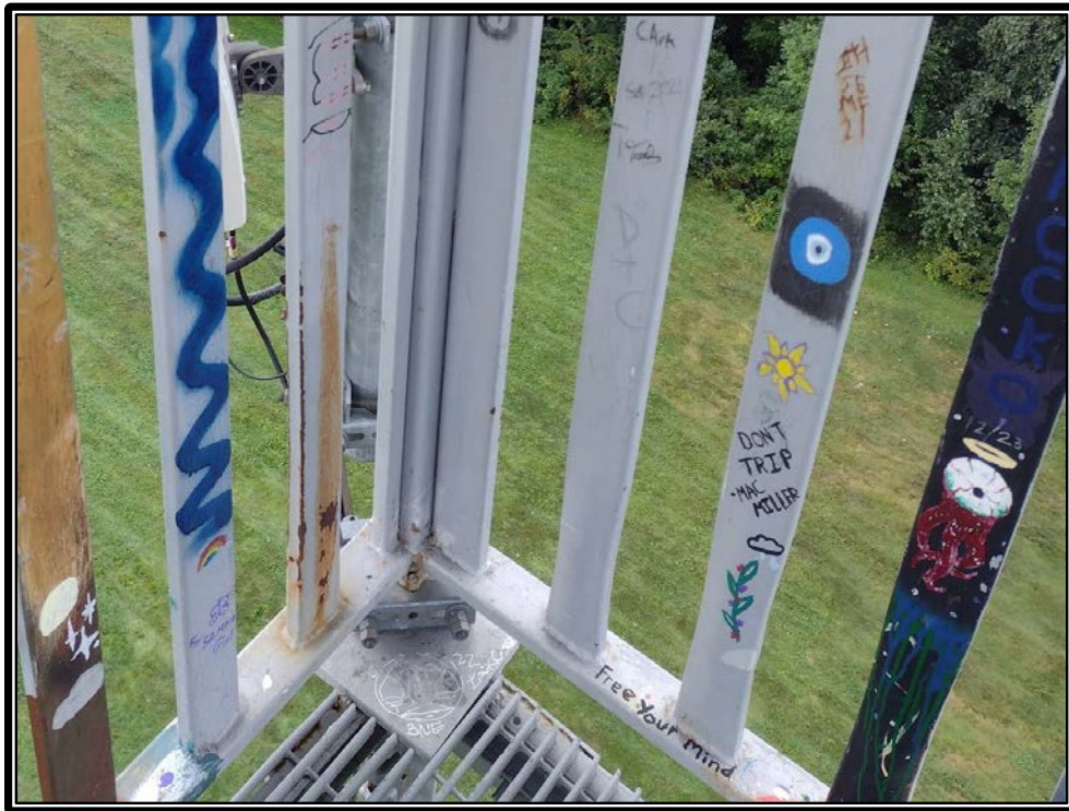
Photo 20: Deformed balusters at top level.
