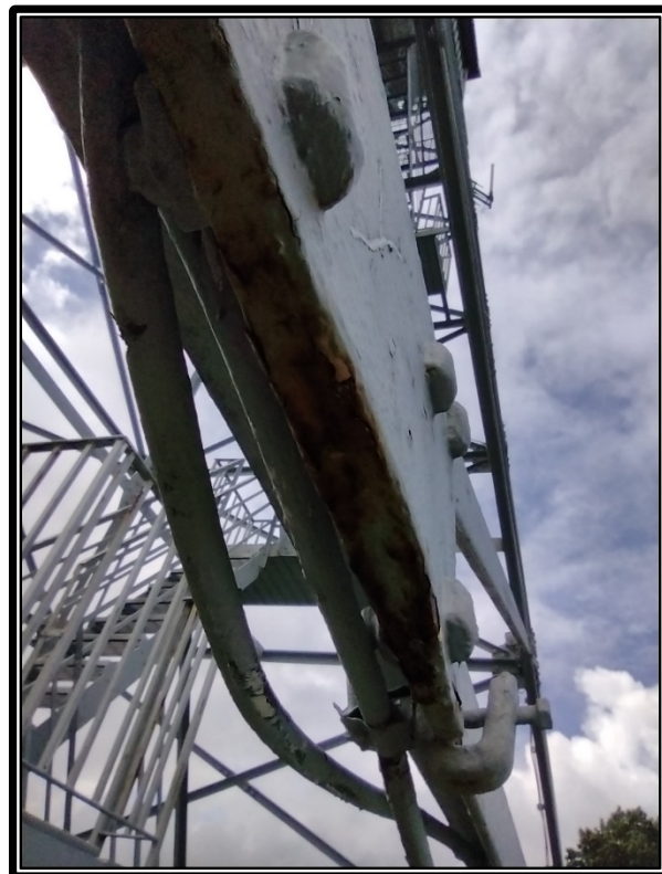
Photo 12: Deformed gusset plate at first level connection.
