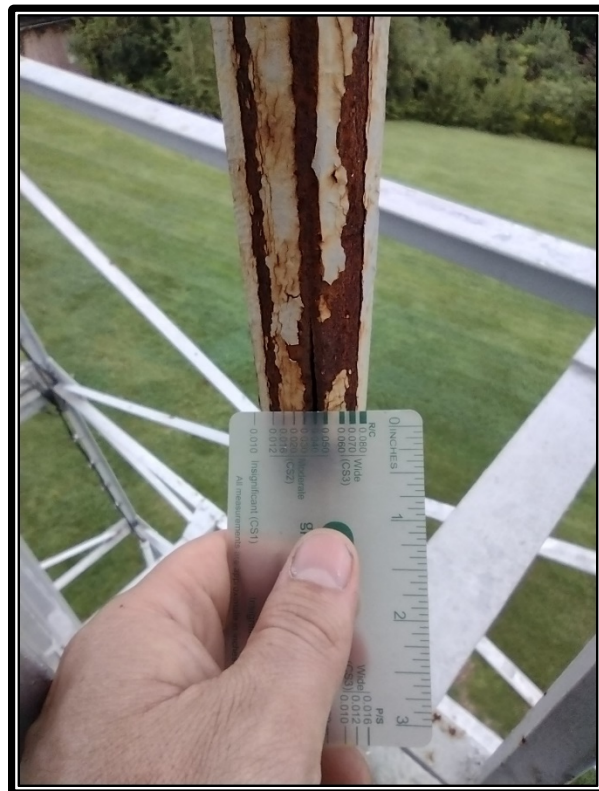
Photo 18: Cracked baluster.
